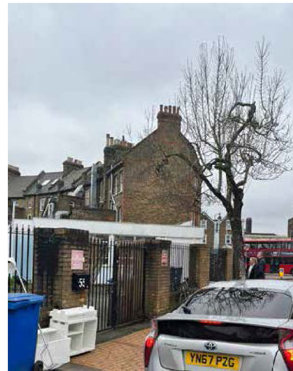
Railings and gables on south boundary
