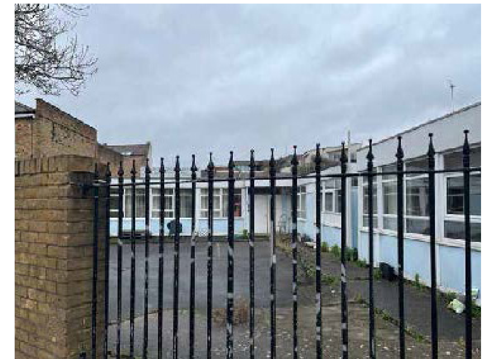
Southern frontage on Nigel Road
